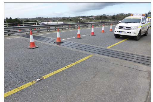
Completion of replaced expansion joint
