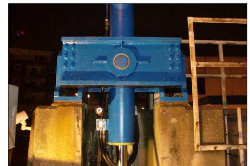
Portsmouth Ferry Port - New gimbal installed
