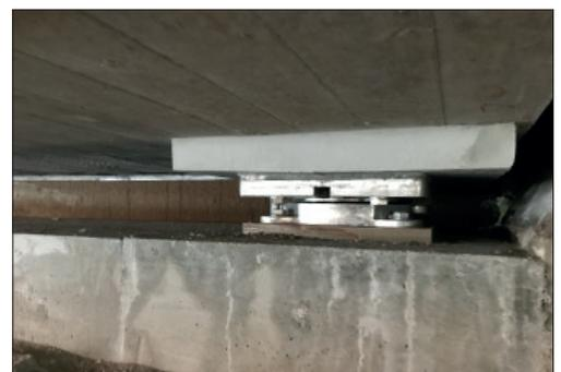
New installed pot bearing
