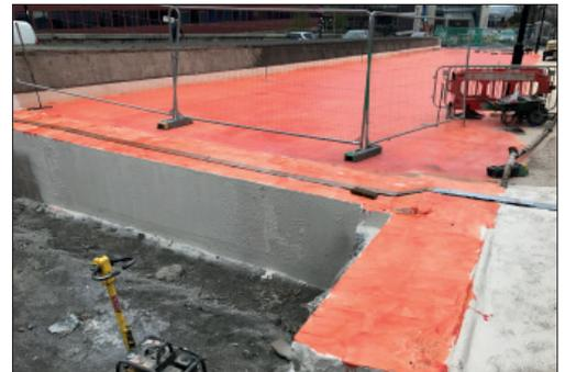
Water proofing applied to the bridge deck
