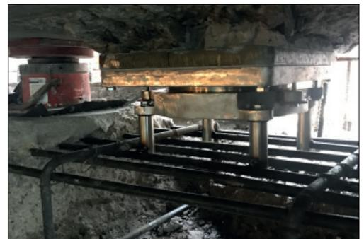
Temporary jacks, hydro demolition and bearing installation
